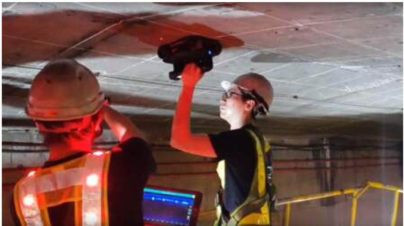
The Proceq GP8000 GPR scanning thick concrete
