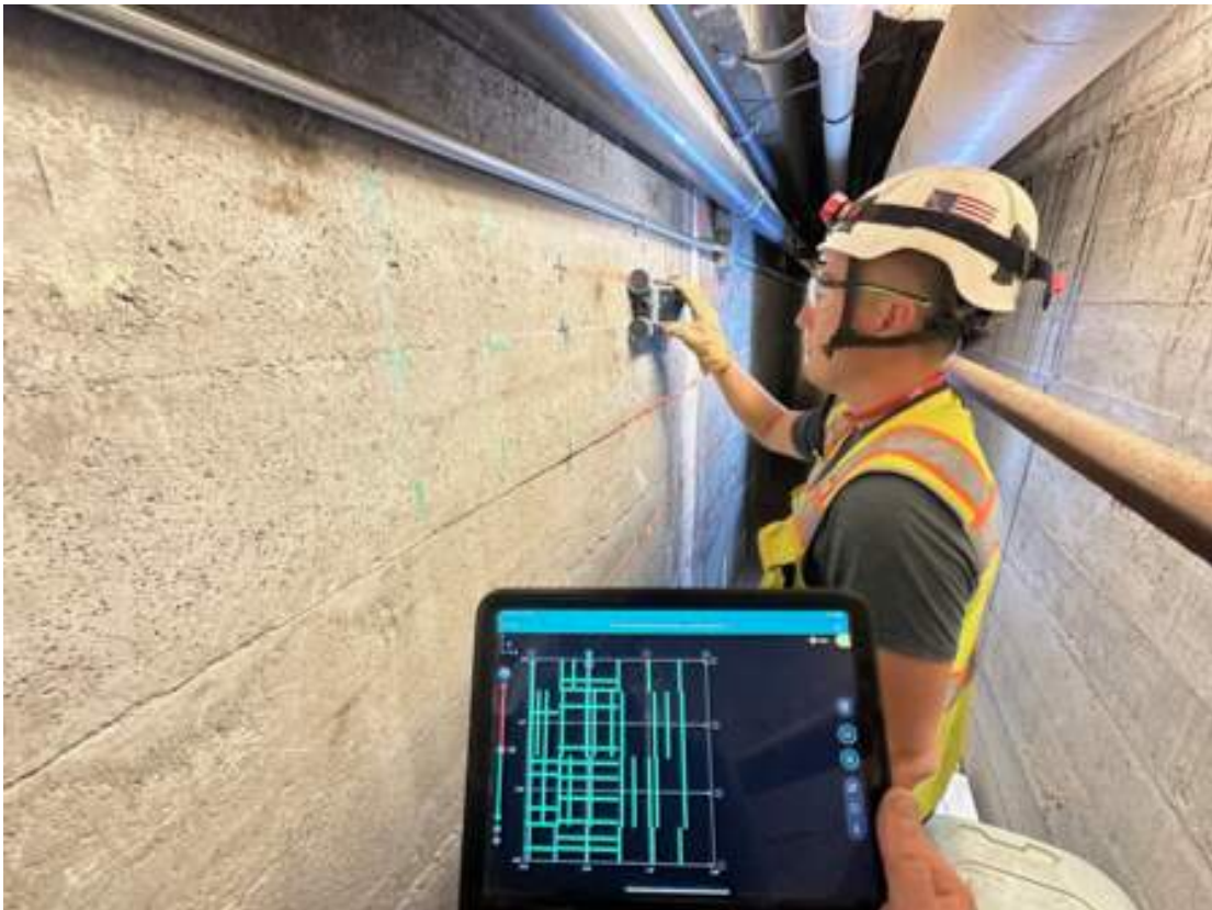
Reinforcement detailing with the Profometer PM8000 Pro cover meter, visualizing the results instantly on the iPad
