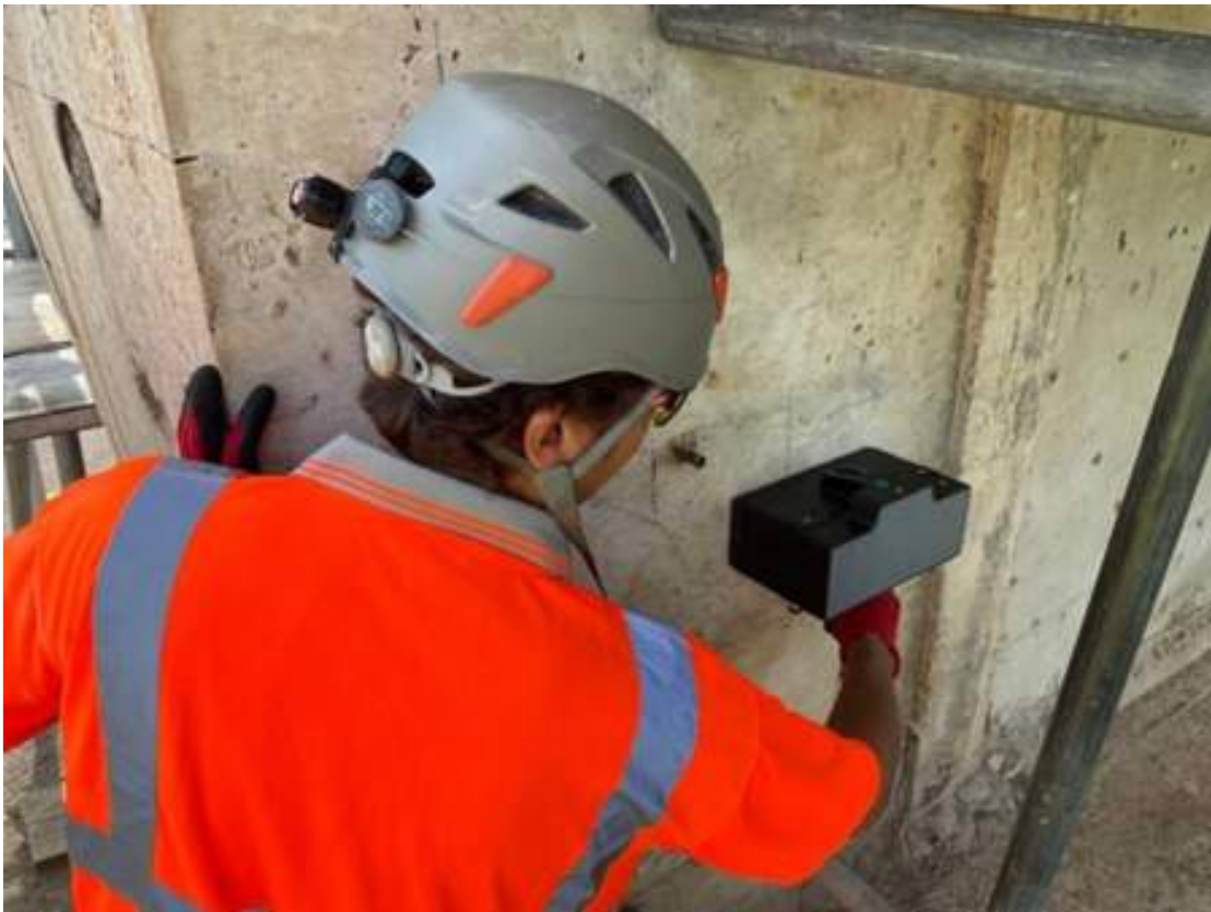
Non-destructive testing on the Huntingdon Railway Viaduct
