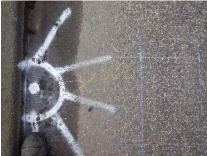
The indicated position for the light poles
