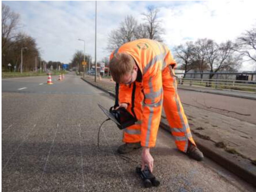
Using the Profometer on the bridge
