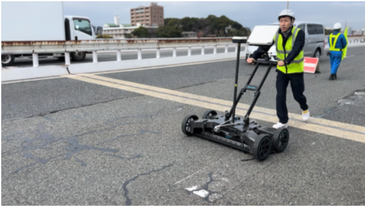
The GS9000 scanning the Fukuoka Expressway in Japan
