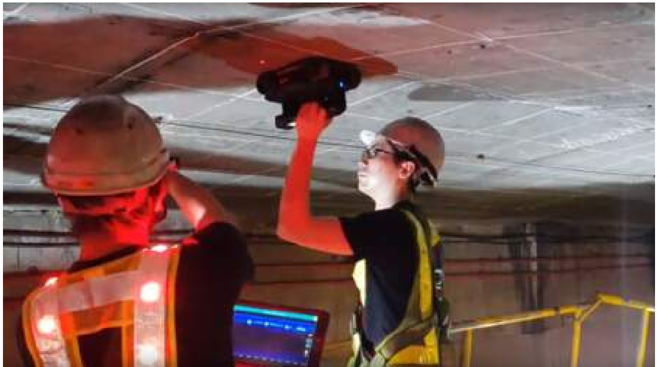
The Proceq GP8000 GPR scanning thick concrete
