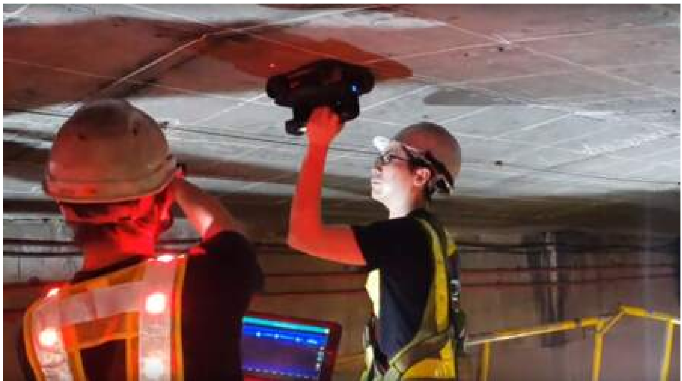
The Proceq GP8000 GPR scanning thick concrete
