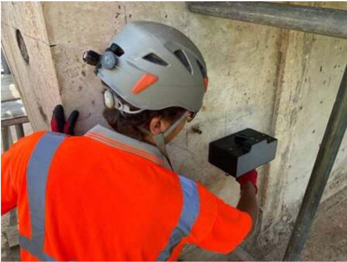
Non-destructive testing on the Huntingdon Railway Viaduct
