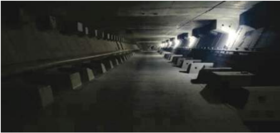
Figure 1. PT tendon locations inside the box beam
