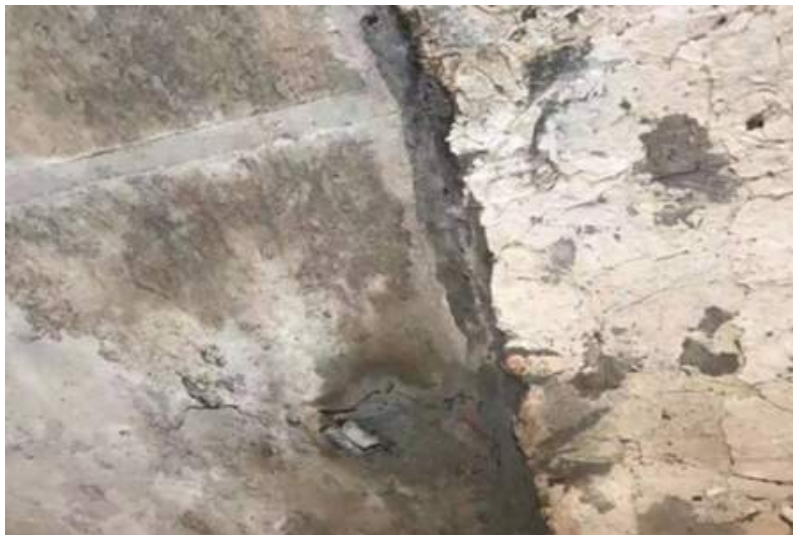
Undamaged areas (back plate)
