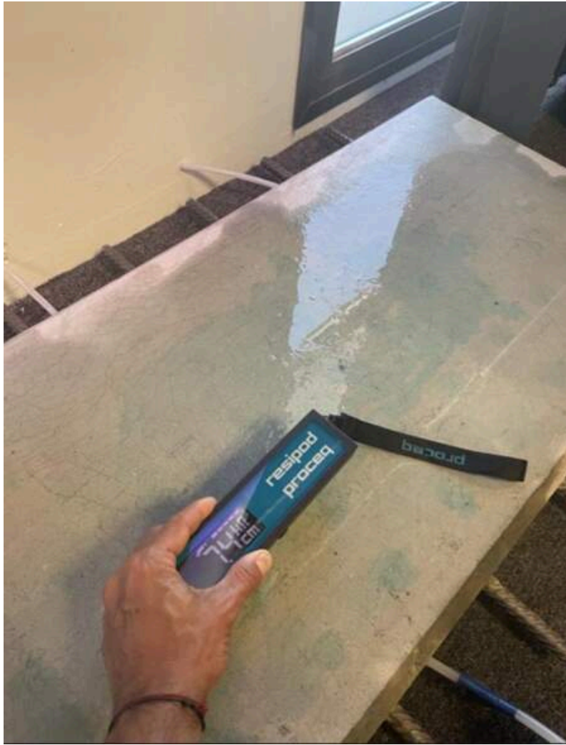
Concrete resistivity results using Resipod
