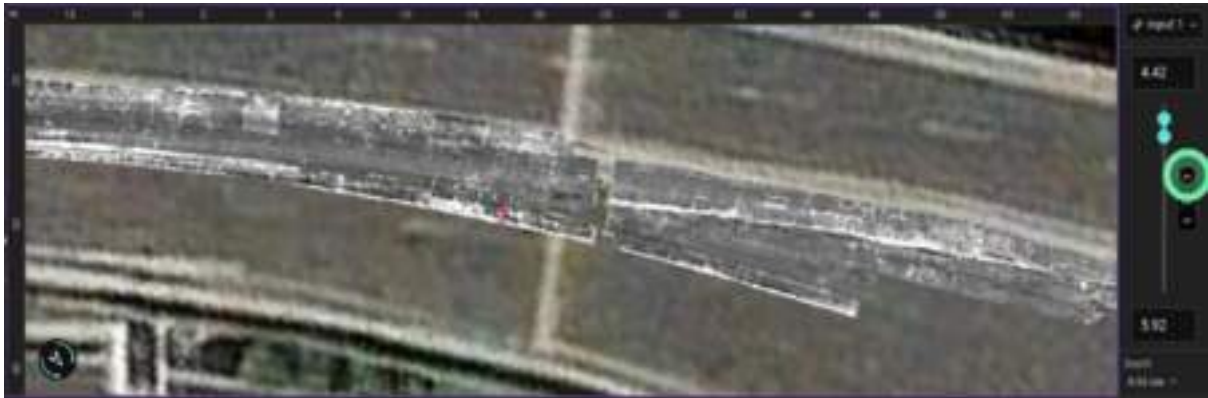
Figure 6. Extended surface layer defects were found at depths of 4 to 6 cm within the asphalt layer.
