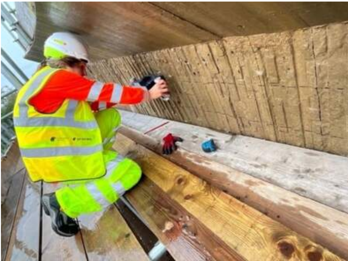
The Pundit PD8050 being used to detect hidden voids in the concrete.
