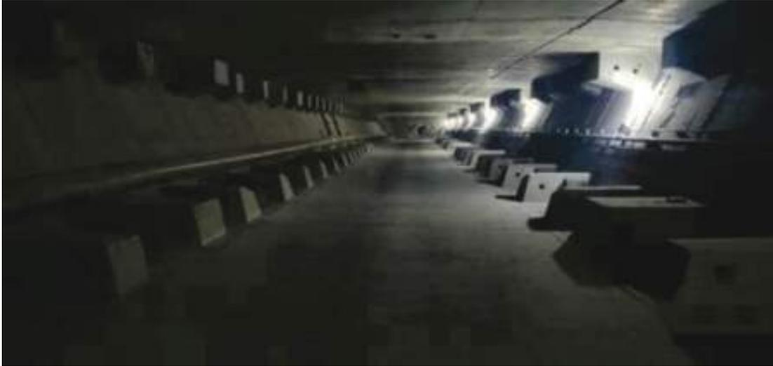
Figure 1. PT tendon locations inside the box beam
