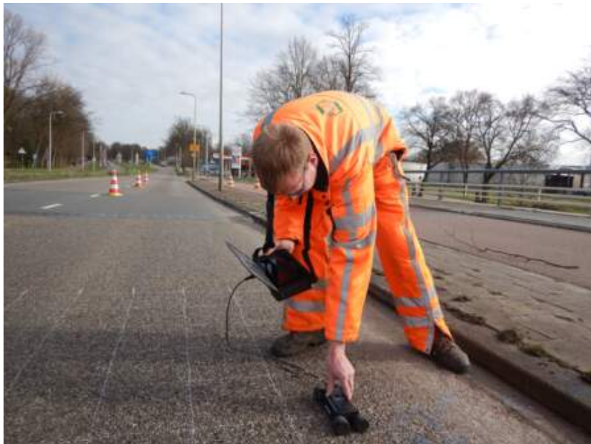
Using the Profometer on the bridge
