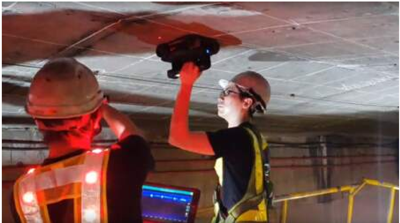
The Proceq GP8000 GPR scanning thick concrete
