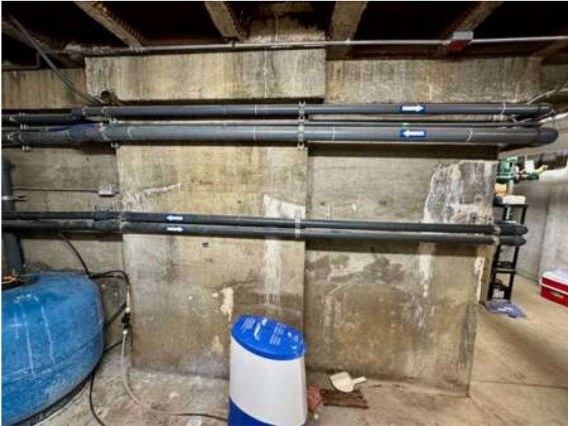
Significant areas of the concrete were compromised, and the steel reinforcement showed signs of corrosion. This deterioration posed risks to safety and operational efficiency, necessitating a thorough condition assessment to determine the appropriate remedial measures.
