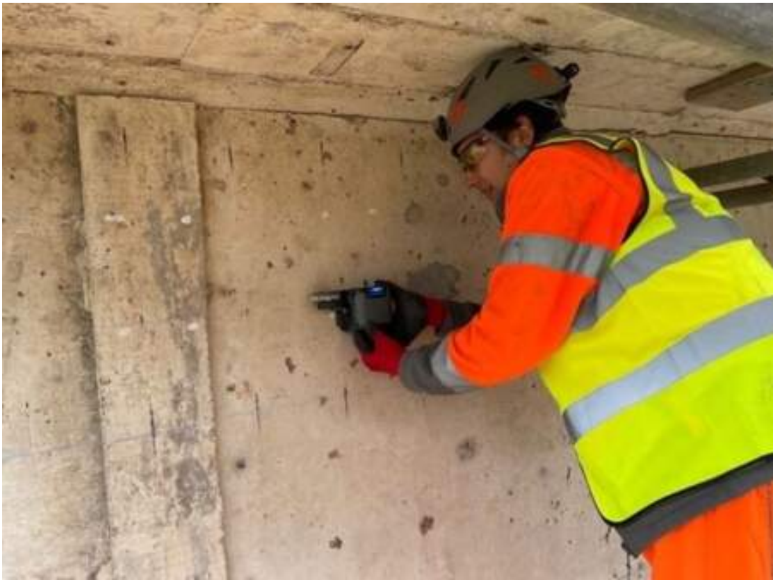
The Proceq GP8800 GPR being used to locate the post-tension ducts
