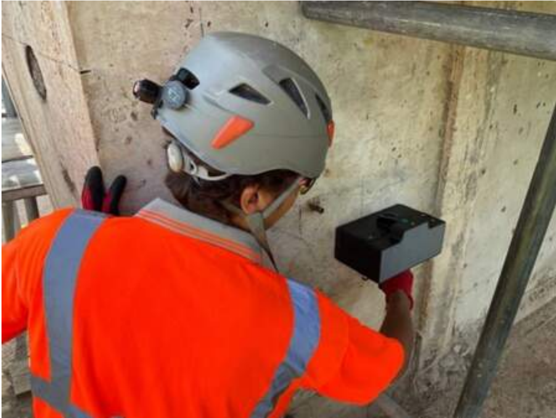
Non-destructive testing on the Huntingdon Railway Viaduct
