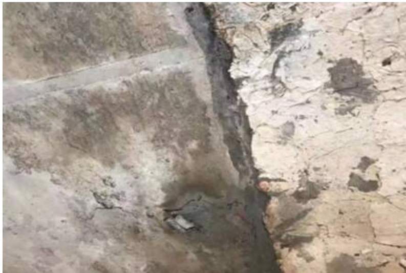
Undamaged areas (back plate)
