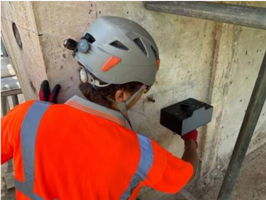
Non-destructive testing on the Huntingdon Railway Viaduct
