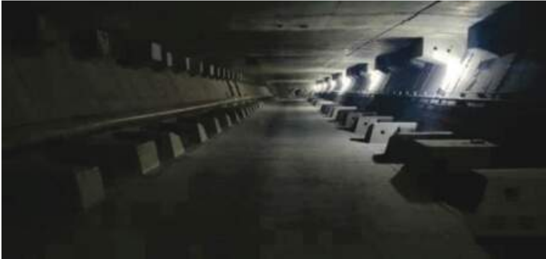
Figure 1. PT tendon locations inside the box beam
