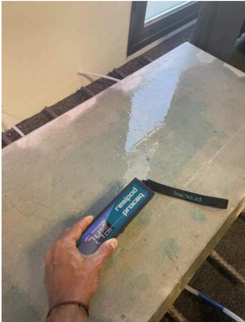
Concrete resistivity results using Resipod
