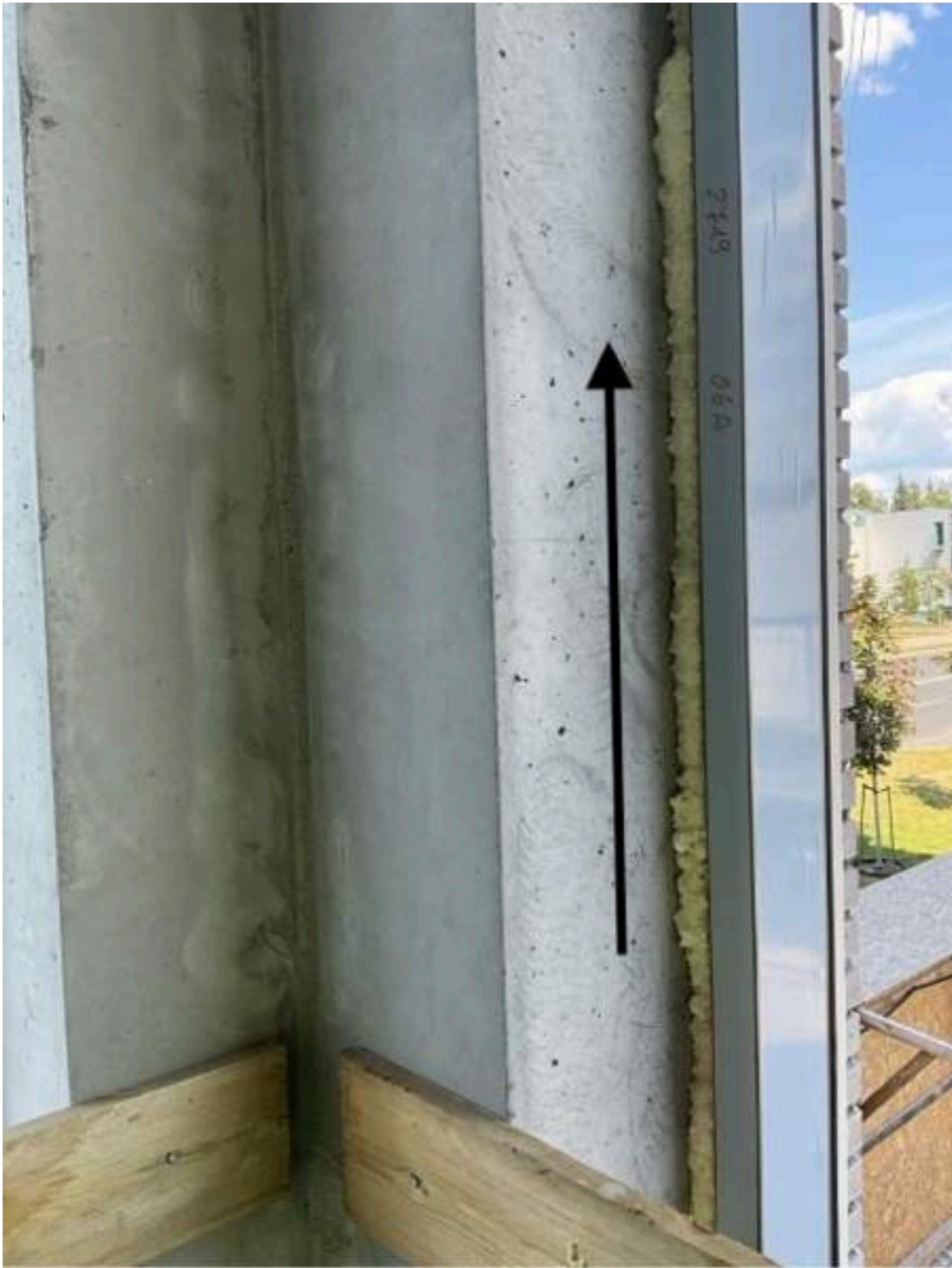
The black arrow shows the direction of the scan along the window reveal.
