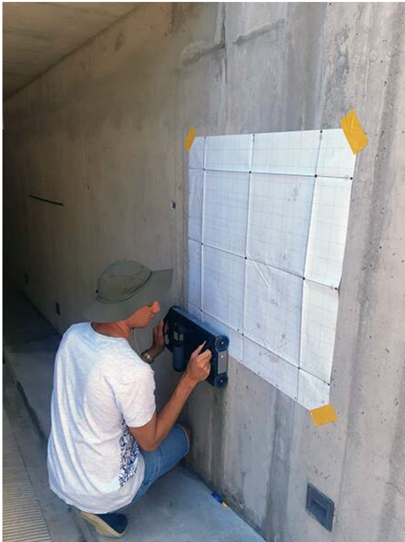
Using the GP8100 to collect an area scan
