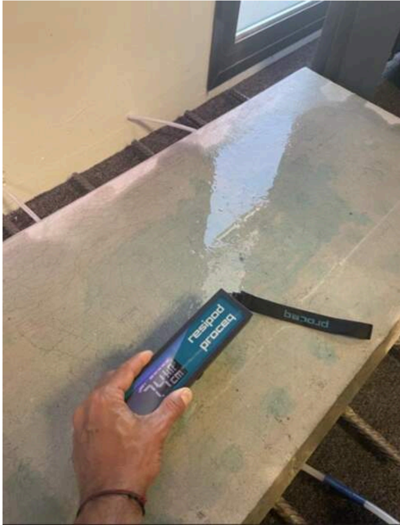
Concrete resistivity results using Resipod
