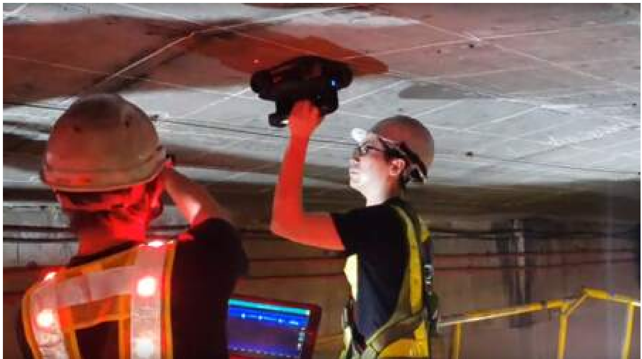
The Proceq GP8000 GPR scanning thick concrete
