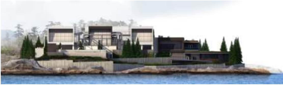
Image source: https://www.hdrinc.com/ca/portfolio/mcloughlin-point-wastewater-treatment-plant
